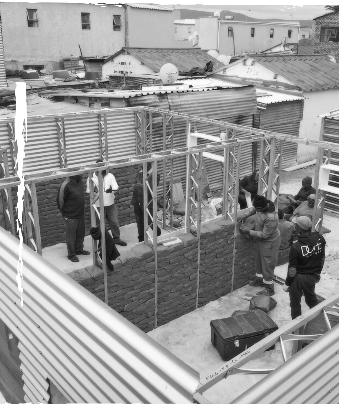
The use of local labour in building sandbag houses in Mshini Wam, Cape Town. Image courtesy of UBU.
