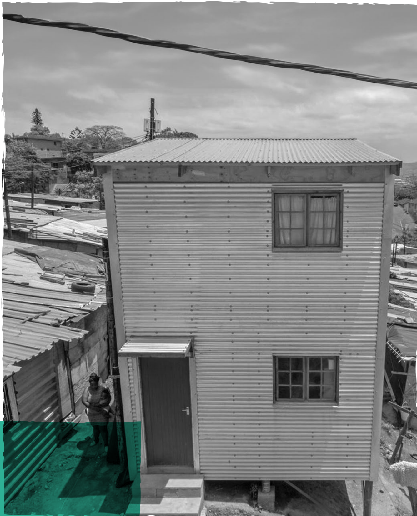
LIFT house, eThekweni. Image courtesy of PPT.
